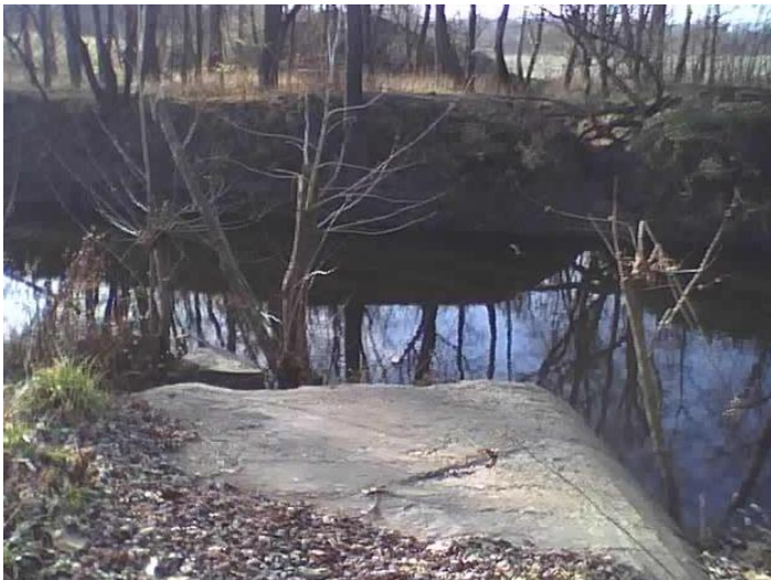
Rt-66 bridge foundation at east bank of Macoupin Creek.
