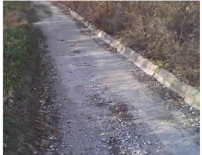
Rt-66 original pavement east of Macoupin Creek. Note roadside berm.
