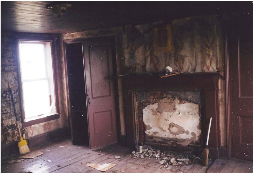
East end ground floor kitchen. Doors are storage cabinets.
