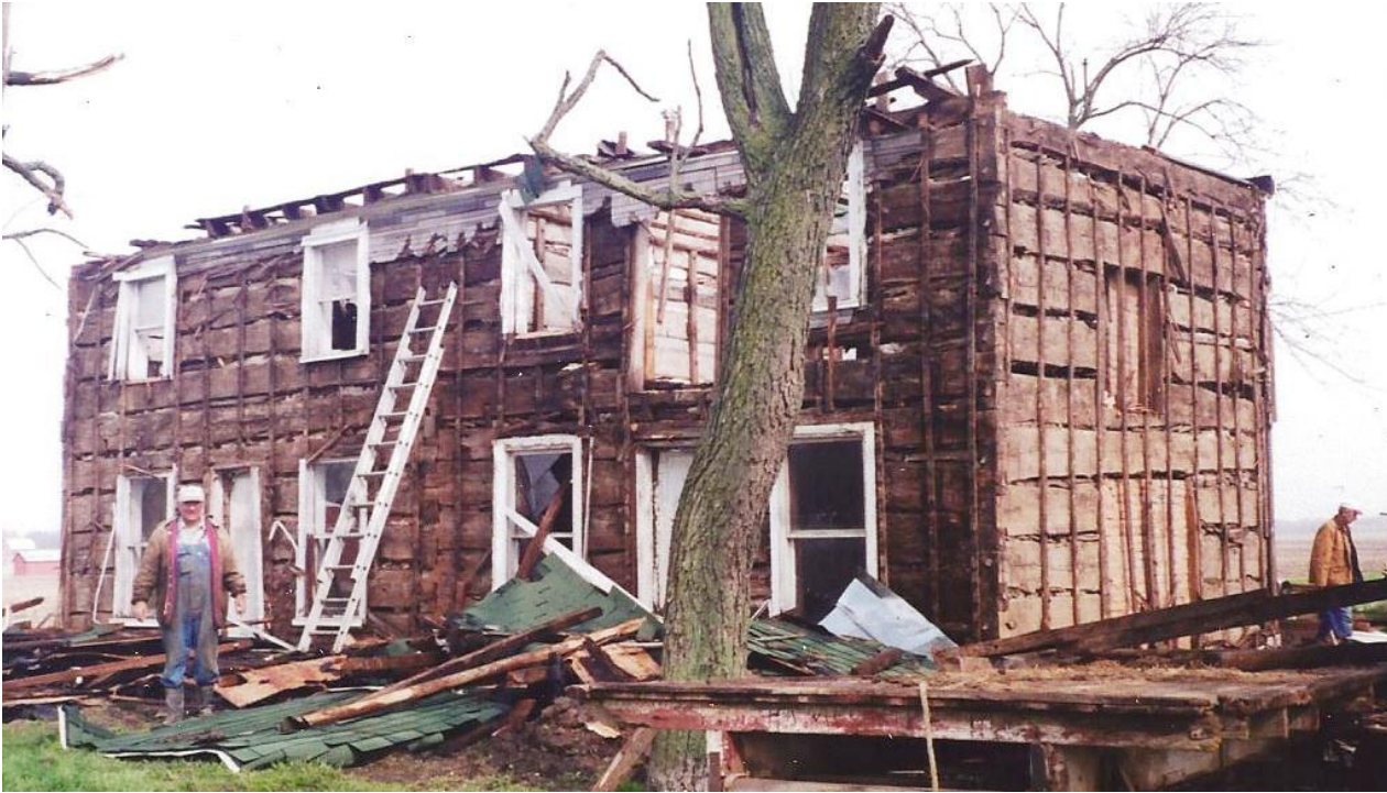
Modern exterior weather-proofing and window removal. Doorway on 2 nd floor is visible. It's outside stairway is not recovered, and it is uncertain if it ascended to the east or west.
