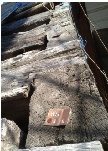
View from ground level looking straight up, depicting coded tags used to facilitate reassembly of logs. Note the log-end “interlock” cut.
