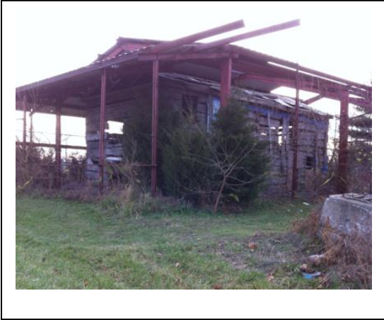
Street view of un-restored inn and partially-built protective structure.
