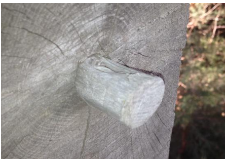
Hewn log end showing construction peg originally used only to secure window frames to hewn logs.
