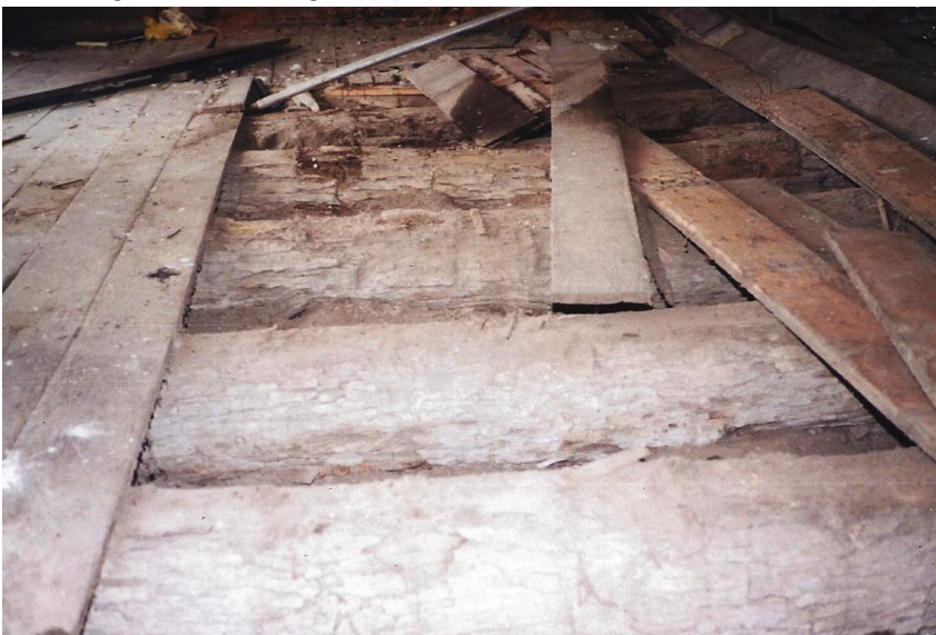
Un-hewn, 17" diameter ground floor support logs are original and weigh ~1,435 lbs each. They had to be pried out of the host earth.
